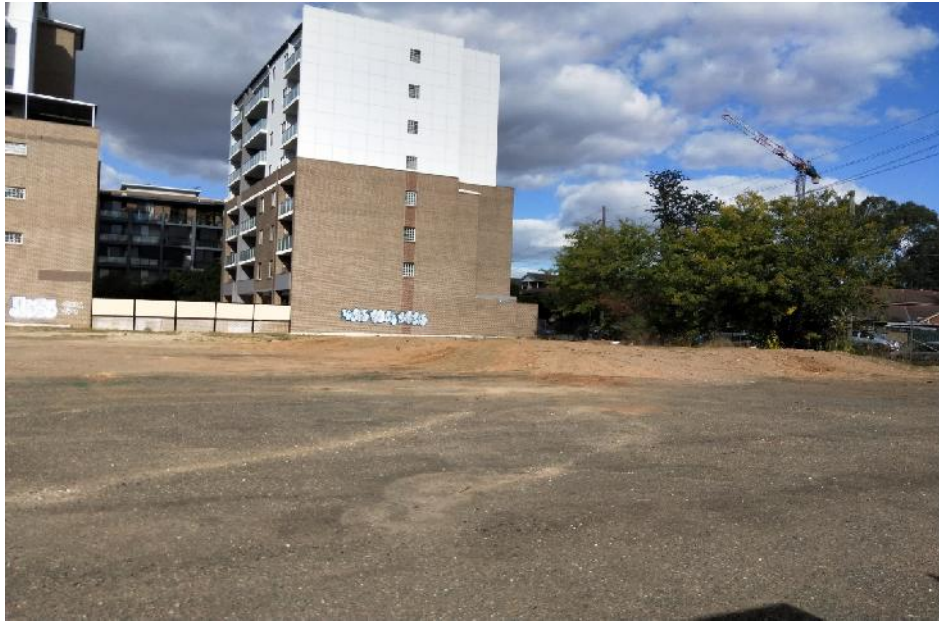
Photo 1 - Spoil stockpile on the southern end of the site
