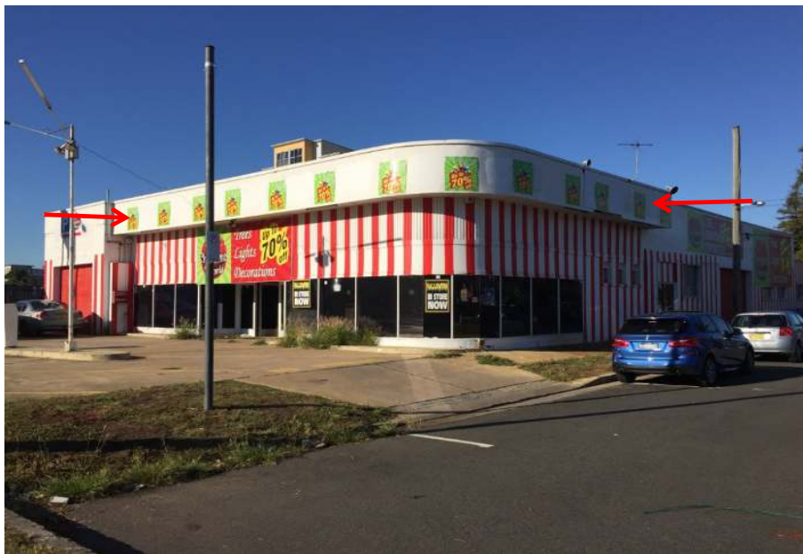
Photograph 2: Main Building, exterior, north and west, upper fascia lining to showroom, fibre cement sheeting, no asbestos detected by analysis
