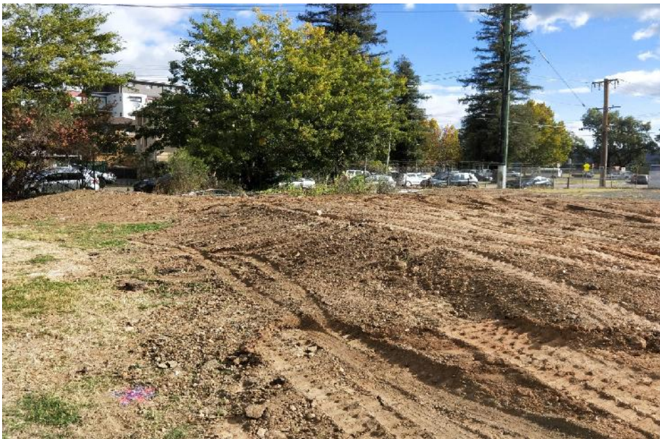
Photo 2 - Spoil stockpile on the southern end of the site
