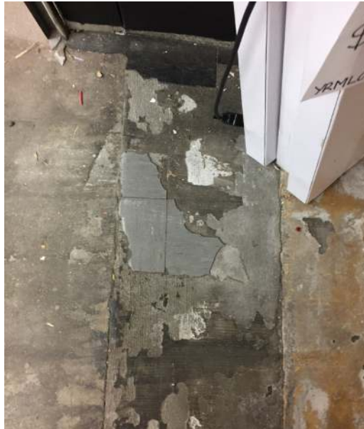
Photograph 28: Main Building, interior, northern entrance, floor adjacent eastern roller door, remnant grey vinyl tile, no asbestos detected by analysis.
