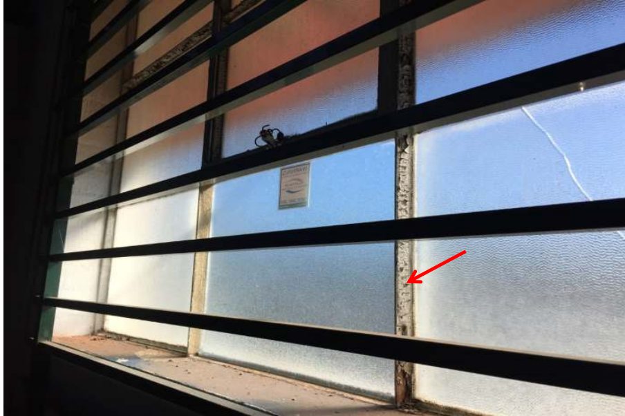
Photograph 45: Main Building, interior, main warehouse area, southwest corner, steel window frame, glazing putty, no asbestos detected by analysis.
