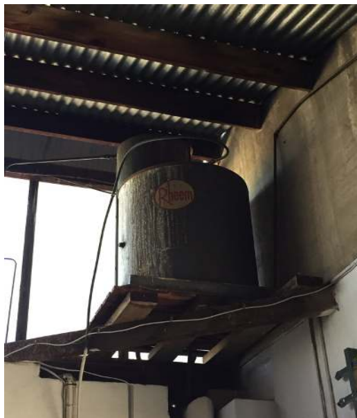
Photograph 37: Main Building, interior, main warehouse, southwestern corner, hot water unit, primary insulation material, SMF identified visually
