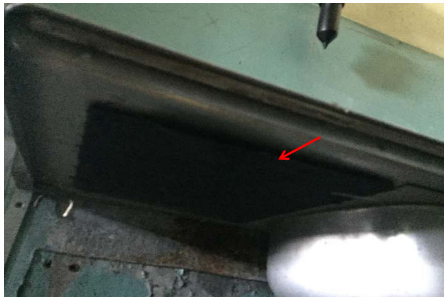
Photograph 48: Main Building, interior, southwestern toilets, sink in northeast corner, bituminous lining, no asbestos detected by analysis
