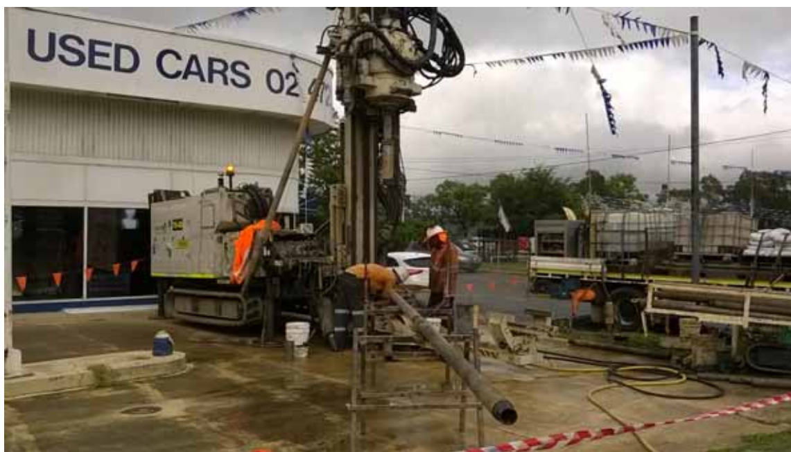
Photo 15 - Drill rig near corner of High and Joh Tipping Grove
