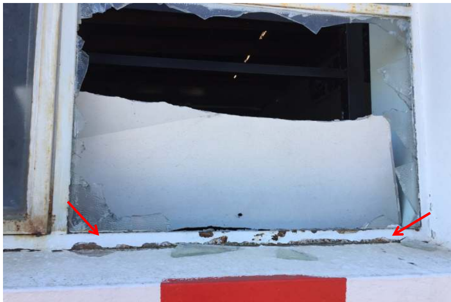
Photograph 12: Main Building, exterior, west, metal window frames, white paint, non-lead paint ( \leq 0.1\% lead w/w).
