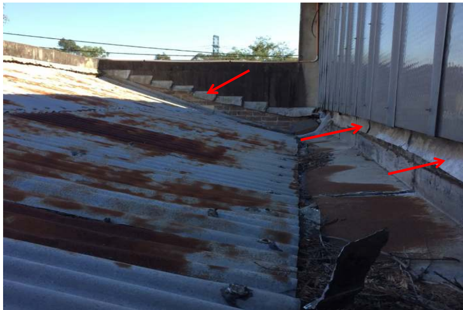
Photograph 26: Main Building, exterior, roofs in general, building joints, flashing, generally assumed lead.
