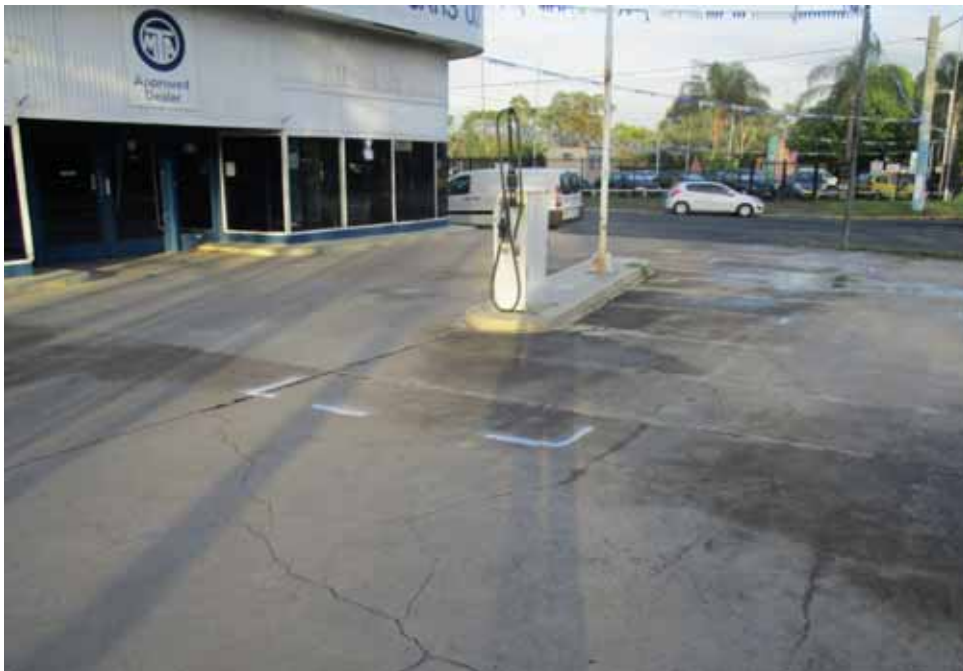
Photo 10 - Marking of UST locations on High Street
