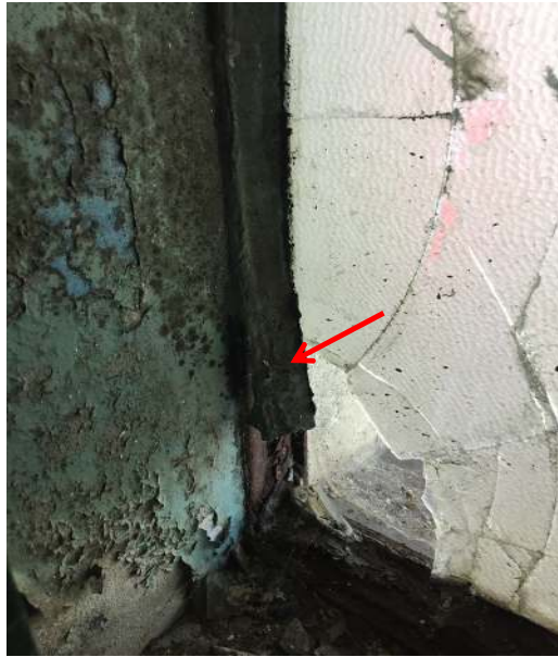
Photograph 49: Main Building, interior, southwestern toilets, interior window, glazing putty, no asbestos detected by analysis
