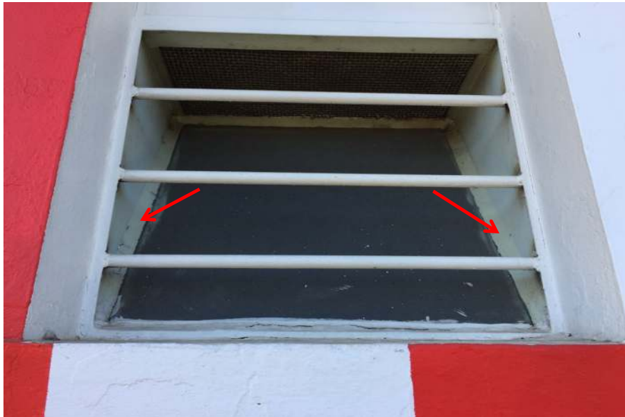
Photograph 8: Main Building, exterior, west, amenities windows, glazing putty, no asbestos detected by analysis.
