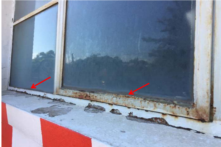
Photograph 11: Main Building, exterior, west, metal window frames (approx. 4), putty, no asbestos detected by analysis.
