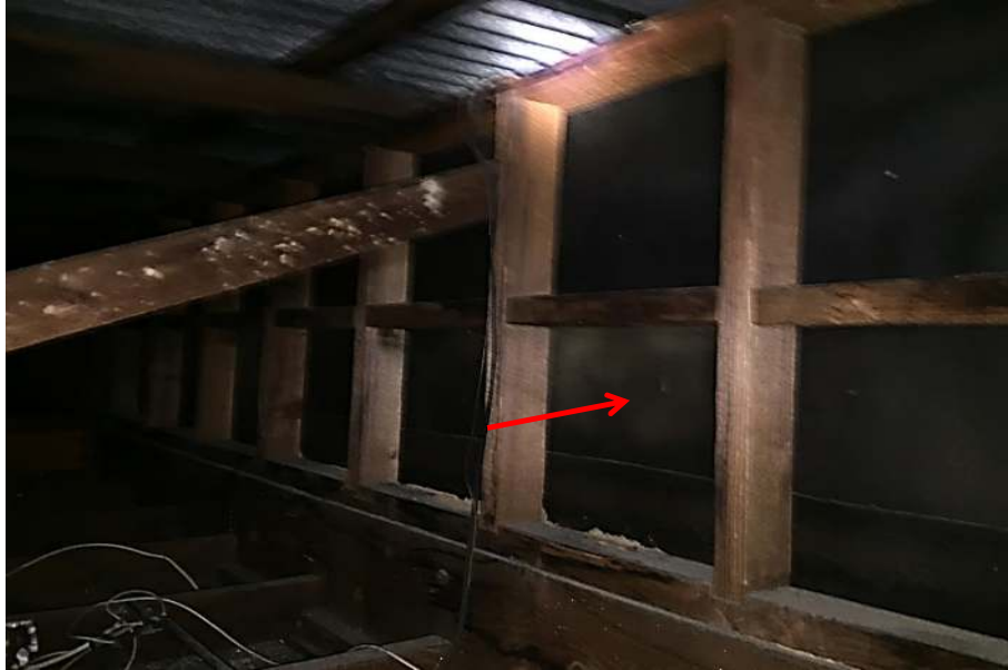
Photograph 43: Main Building, interior, northern entrance, ceiling cavity, bituminous lining to fascia, no asbestos detected by analysis.
