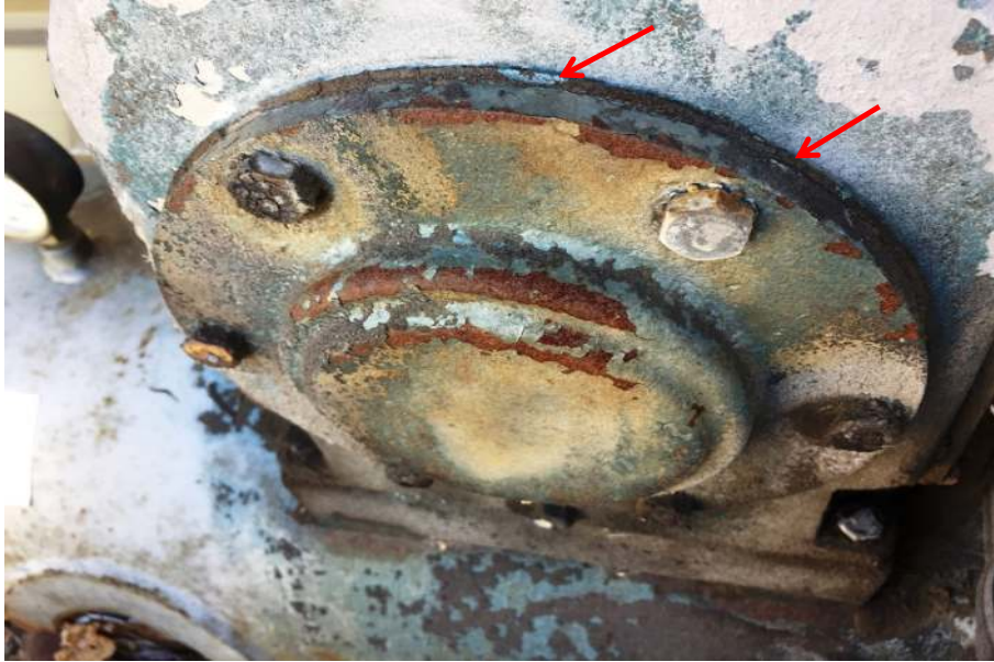
Photograph 23: Main Building, exterior, east, plant, typical gasket, no asbestos detected by analysis.
