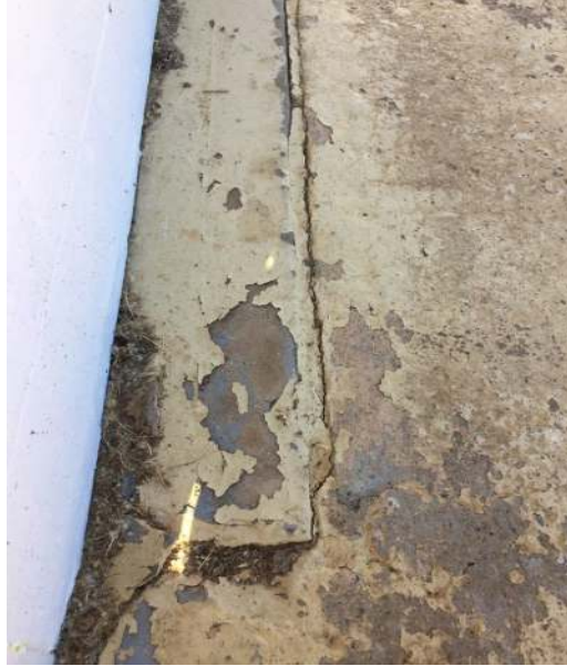
Photograph 7: Main Building, exterior, northwest, hardstand area, brown paint, non-lead paint ( \leq 0.1\% lead w/w).
