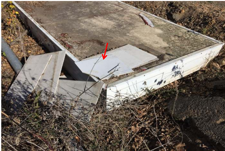
Photograph 50: Exterior grounds, southern end of site, ground surfaces, fibre cement board, no asbestos detected by analysis
