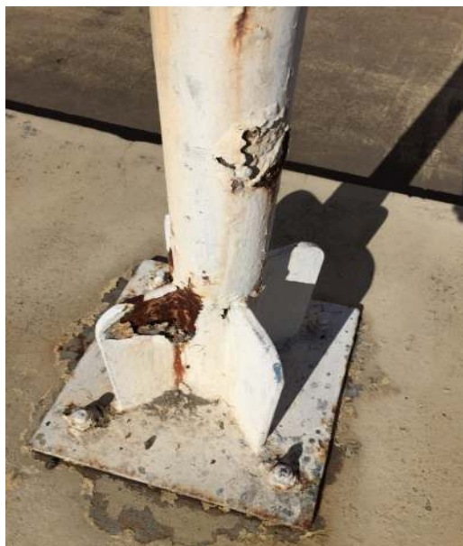
Photograph 15: Main Building, exterior, north, light pole, white paint, non-lead paint ( \leq 0.1\% lead w/w).
