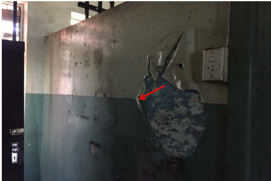
Photograph 46: Main Building, interior, southwestern toilets, typical wall, olive green and white paints, non-lead paint ( \leq 0.1\% lead w/w)
