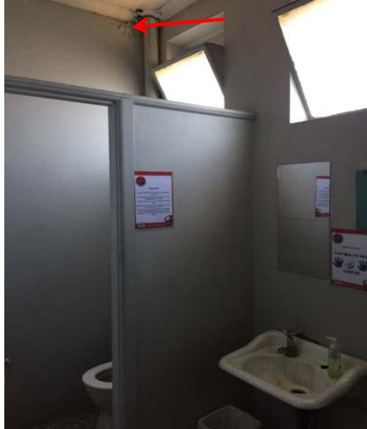
Photograph 31: Main Building, interior, northern entrance area, toilets, typical wall, grey paint, non-lead paint ( \leq 0.1\% lead w/w).
