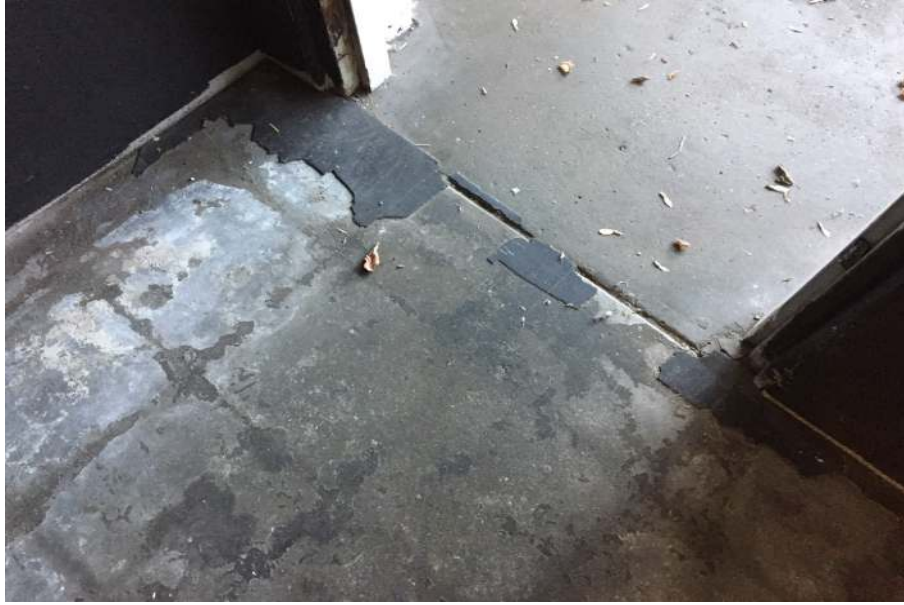
Photograph 29: Main Building, interior, northern entrance, floor near southeast doorway, remnant black vinyl tile, no asbestos detected by analysis.
