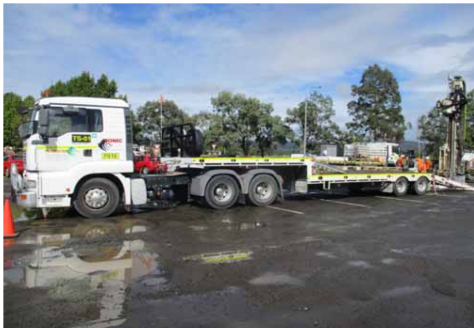
Photo 12 - Drill rig on site in carpark
