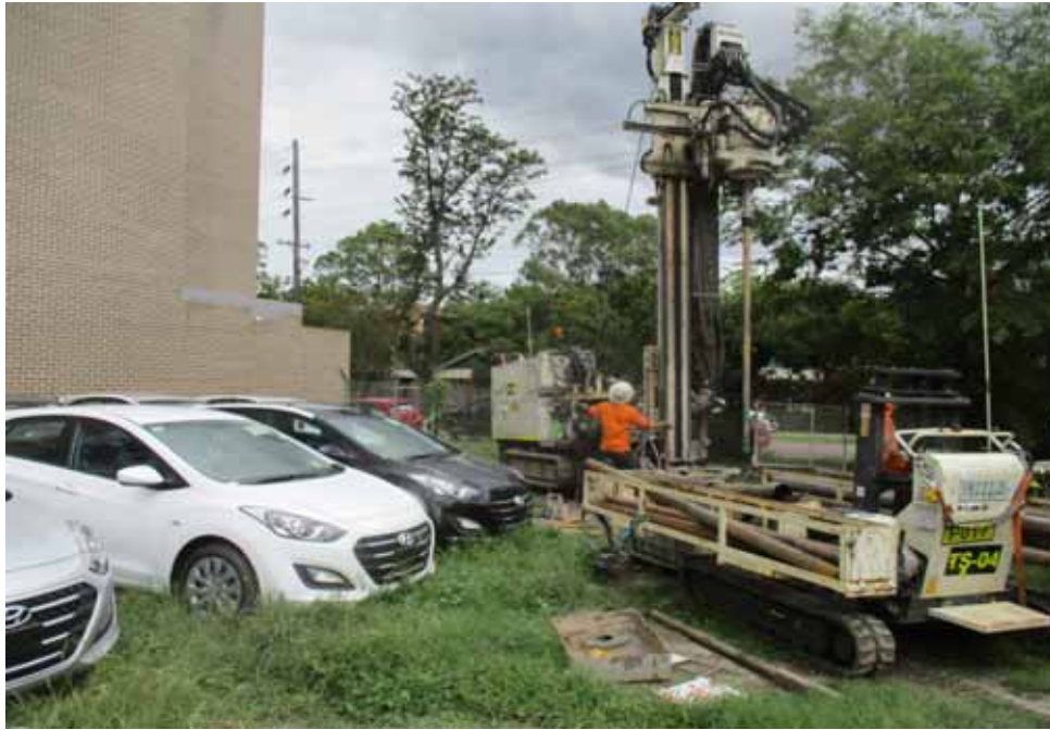
Photo 13 - Drilling operations on unsealed area behind building
