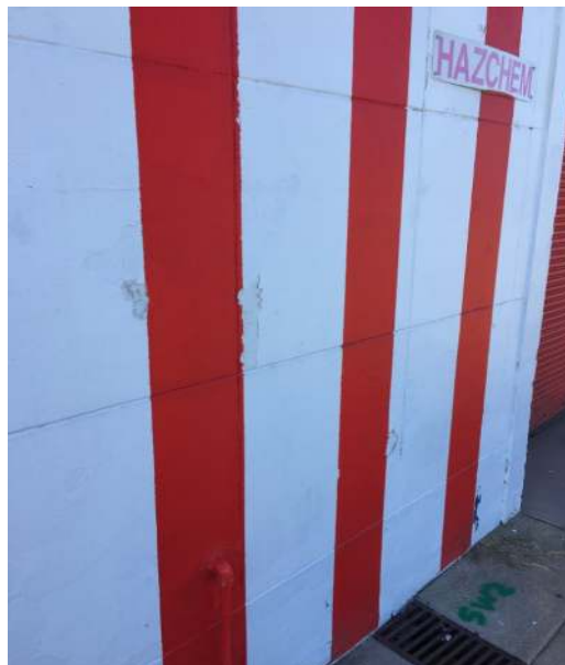
Photograph 10: Main Building, exterior, west, walls, concrete block, white paint, non-lead paint ( \leq 0.1\% lead w/w).
