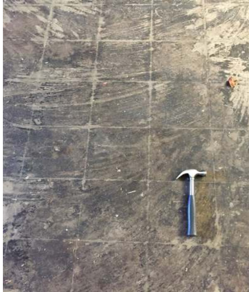
Photograph 27: Main Building, interior, northern entrance, floor generally, bituminous adhesive (previous area of smaller gauge tiles), no asbestos detected by analysis.
