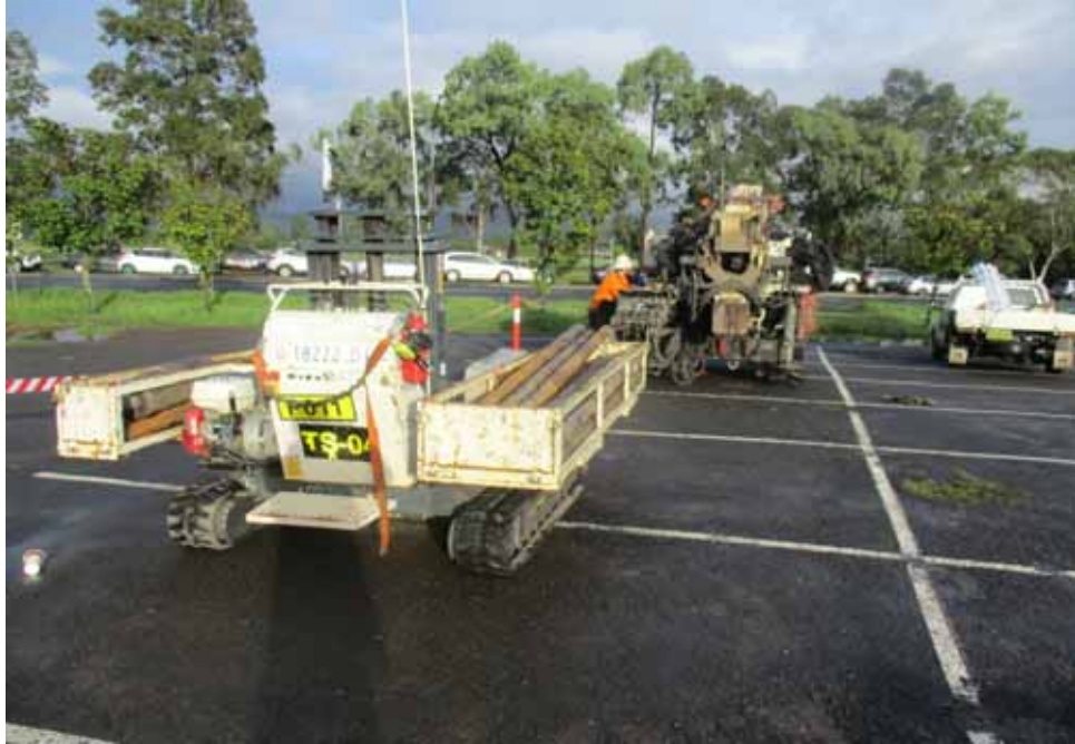
Photo 11 - Drill rig on site in carpark
