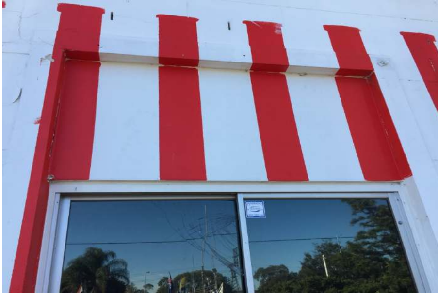
Photograph 9: Main Building, exterior, west, head lining above sliding entrance door, fibre cement sheeting, no asbestos detected by analysis.
