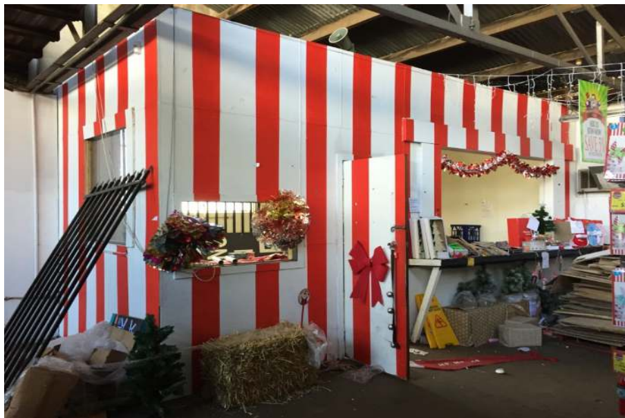
Photograph 34: Main Building, interior, main warehouse, office area, external wall linings, fibre cement sheeting, no asbestos detected by analysis.
