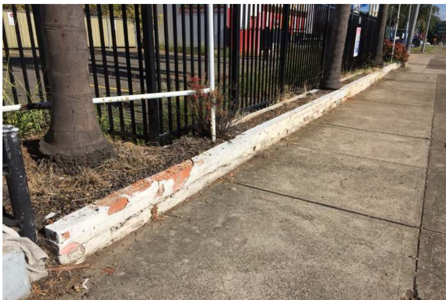
Photograph 16: Main Building, exterior, north, perimeter wall, brick work, white paint, non-lead paint ( \leq 0.1\% lead w/w).
