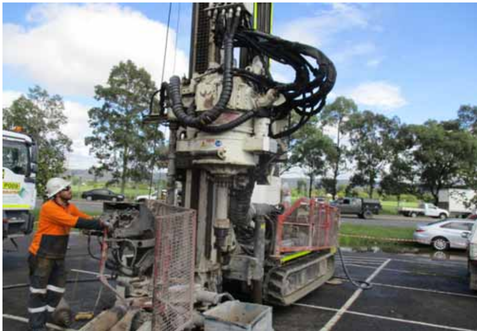
Photo 14 - Drilling underway in carpark
