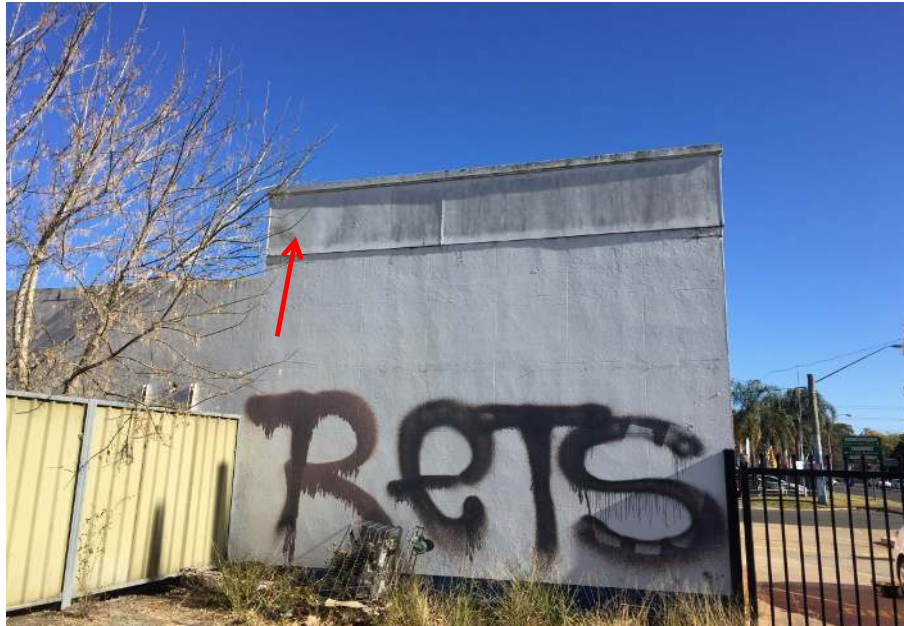
Photograph 1: Main Building, exterior, northeast, head lining to garage generally, fibre cement sheeting, no asbestos detected by analysis
