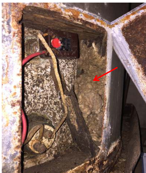
Photograph 56: Main Building, interior, main warehouse, southwestern corner, hot water unit, primary insulation material, SMF identified visually
