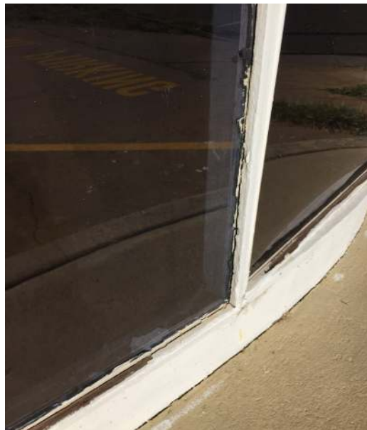
Photograph 6: Main Building, exterior, north, showroom, window frames, white paint, non-lead paint ( \leq 0.1\% lead w/w).
