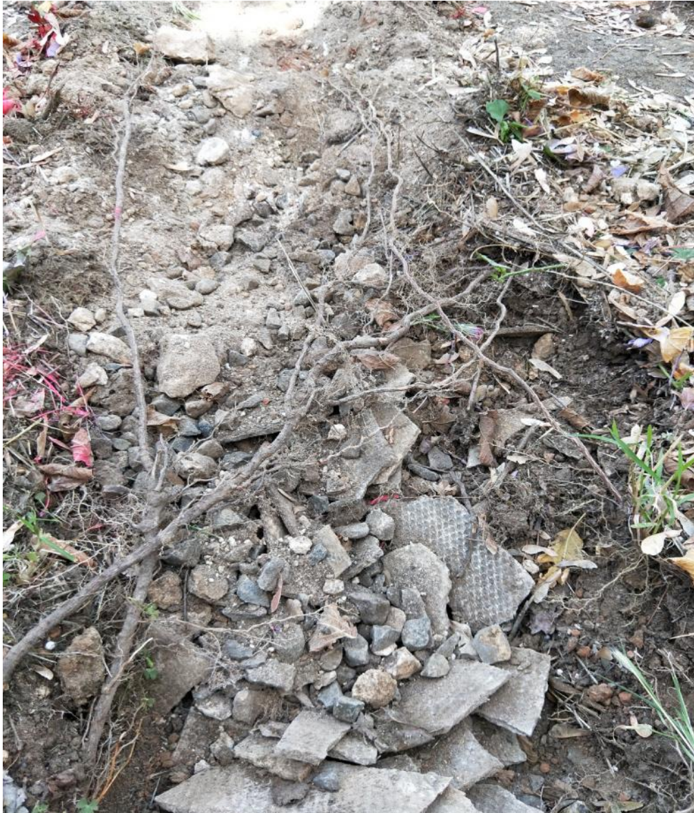
Photo 3 - Fibre cement found at test pit WC18
