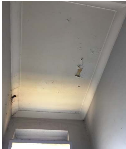
Photograph 32: Main Building, interior, northern entrance area, toilets, typical ceiling, white paint, non-lead paint ( \leq 0.1\% lead w/w).
